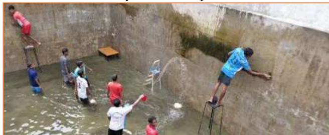
Cleaning of the Water Tank
